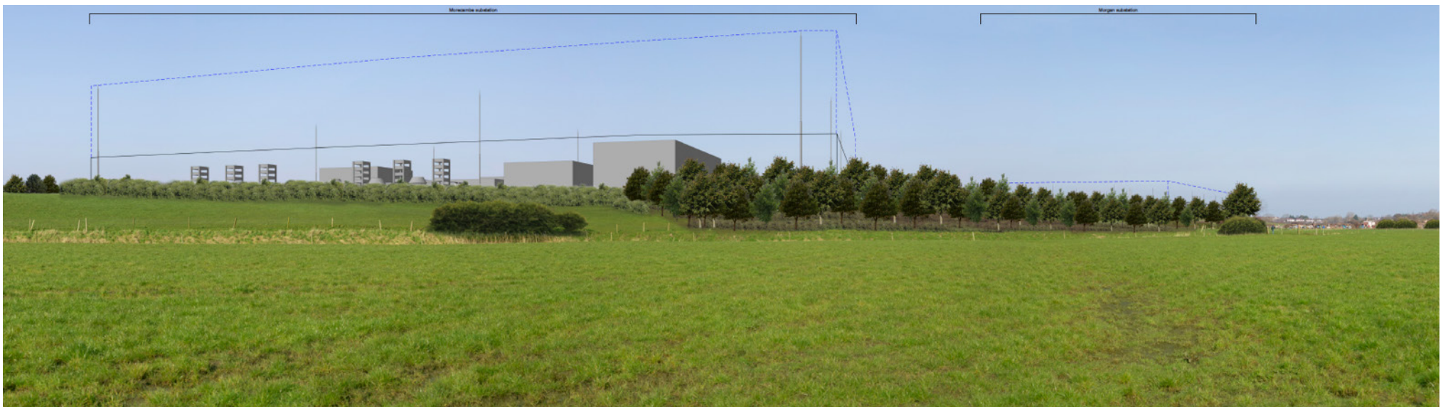
Figure 11: View from footpath north of A584 towards Morecambe substation, showing an indicative layout
